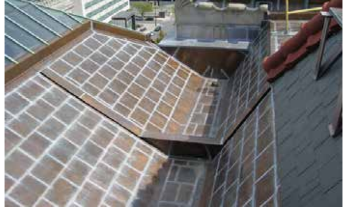
Steep-sloped flat-seam roofing.
