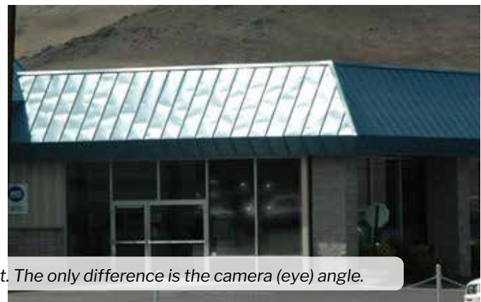
The only difference between invisible (left) and visible (right) oil canning is one hour and the changing of the sun's angle.
